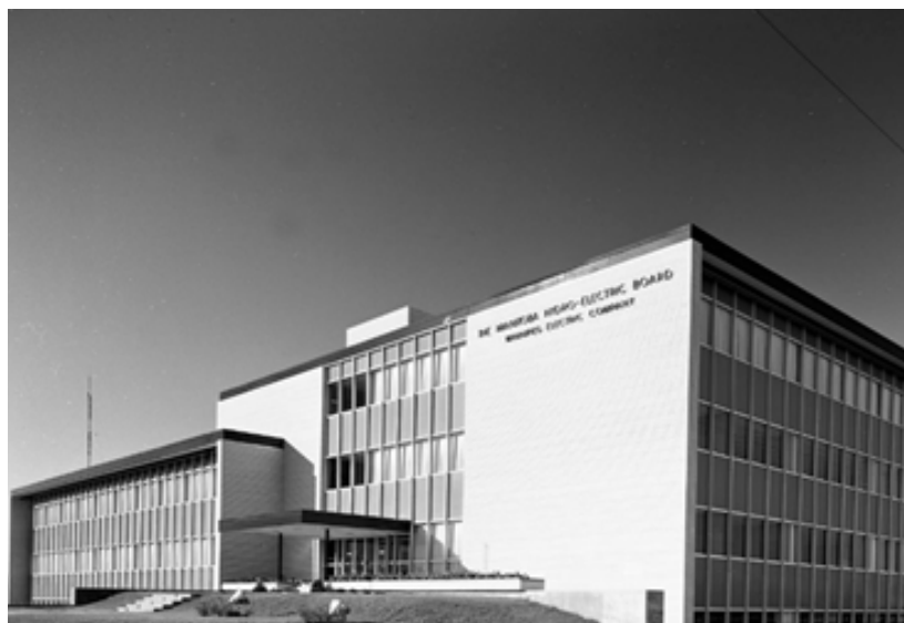
Figure 3: Original Manitoba Hydro-Electric Board building at 1650 Harrow St.
