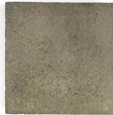
CAST-IN-PLACE CONCRETE FOUNDATIONS & LANDSCAPE STAIRS/LANDINGS
