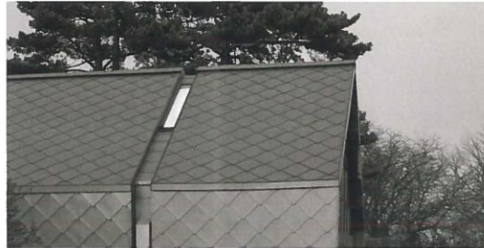
EXAMPLE DIAMOND METAL SHINGLE CLADDING FINISH TO BE IRIDESCENT METAL SHOWN TO THE LEFT IMAGE SOURCE: BACA ARCHITECTS [ https://www.baca.uk.com/amphibious-house.html ]
