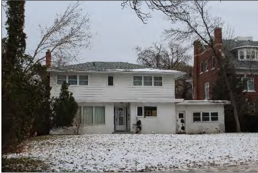
Non-Heritage Building 4 Ruskin Row Built: 1957 Designer: Unknown Contractor: Unknown
