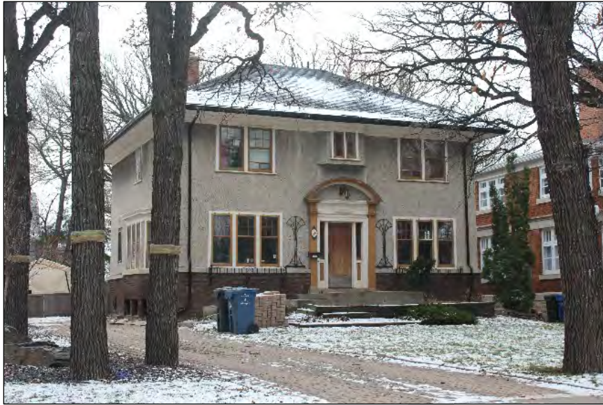
Heritage Building, Principal 66 Harvard Avenue Built: 1925 Designer: Sparrow Brothers (owners) Contractor: Sparrow Brothers (owners) Style: Georgian Revival Influences
