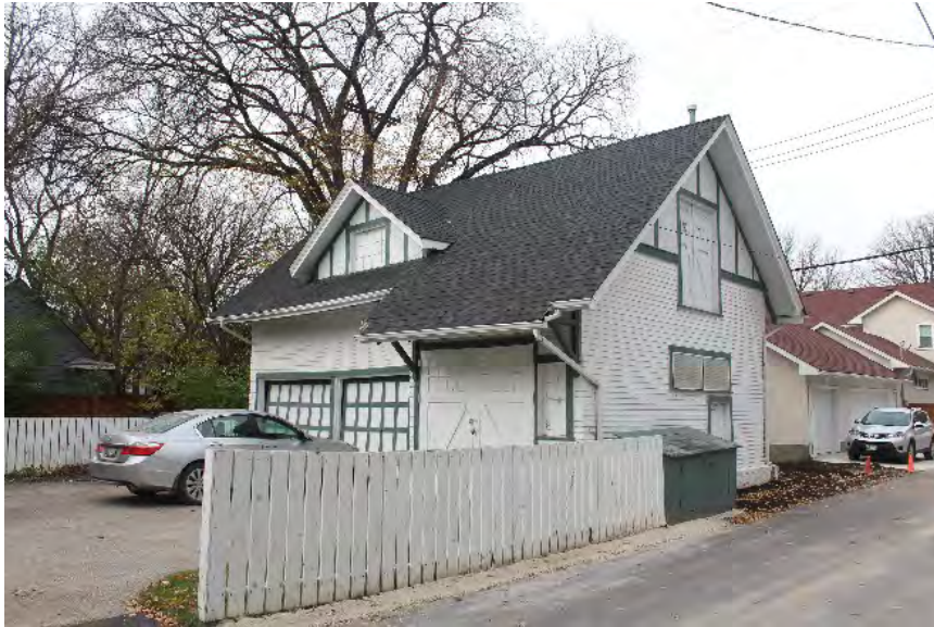
Heritage Building, Accessory 85 Yale Avenue
