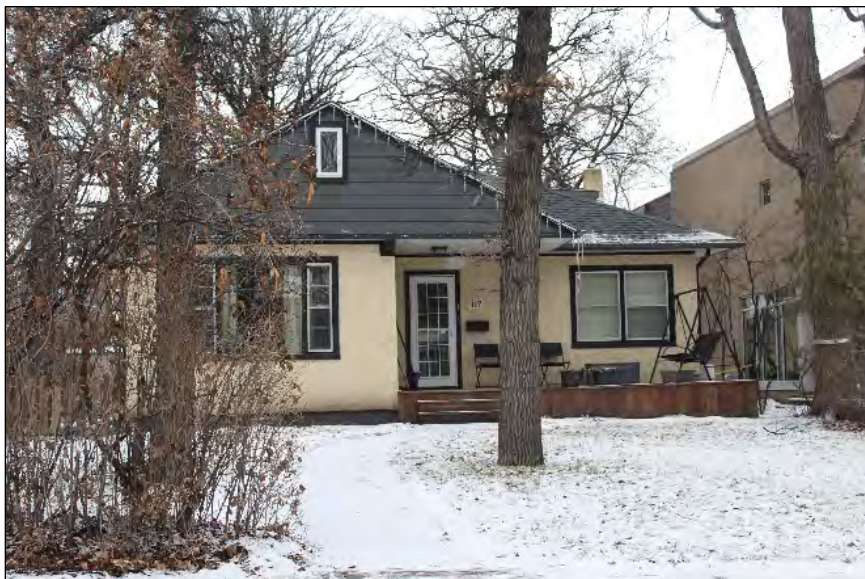
Non-Heritage Building 117 Kingsway Built: 1948 Designer: Unknown Contractor: Unknown
