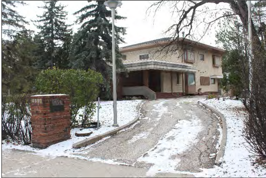
Heritage Building, Principal 456 Wellington Crescent Built: 1977 Designer: IKOY Partnership Contractor: Fuji Builders Ltd. Style: Late Modern/Prairie Style Influences
