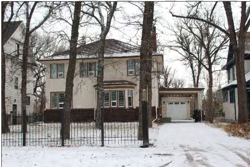
Heritage Building, Principal 101 Kingsway Built: 1927 Designer: Sparrow Brothers (owners) Contractor: Sparrow Brothers (owners) Style: Prairie Style Influences
