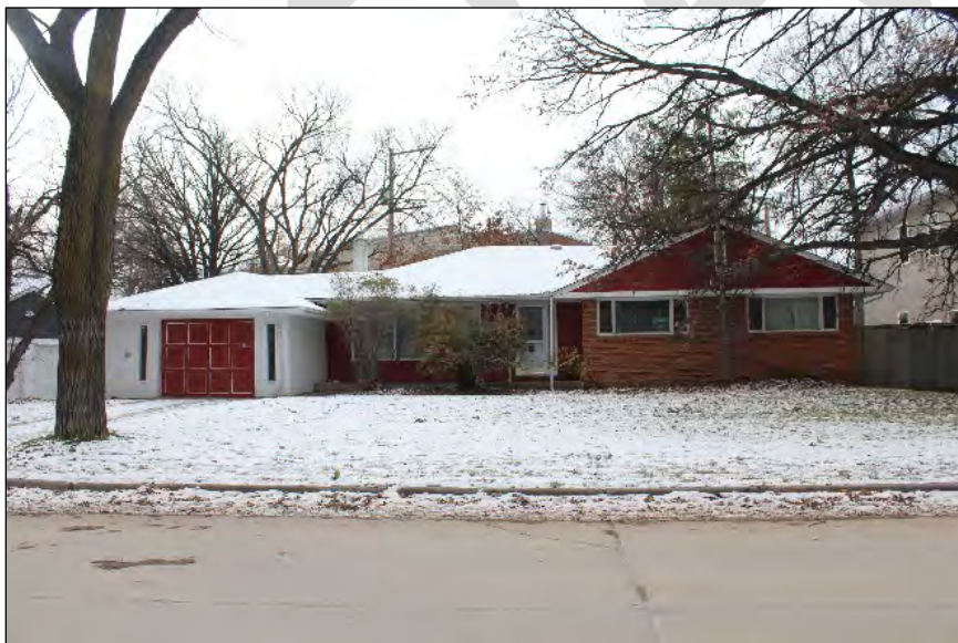
Non-Heritage Building 5 Ruskin Row Built: 1952 Designer: Louis Segal (owner) Contractor: Louis Segal (owner)
