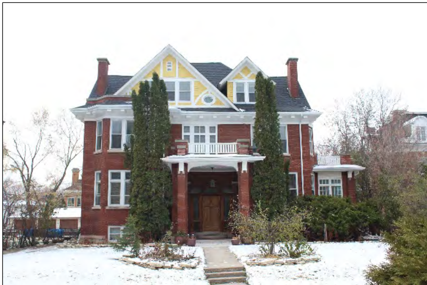
Heritage Building, Principal 412 Wellington Crescent Built: 1906 Designer: H.B. Rugh Contractor: Homes, James & James Style: Queen Anne Revival
