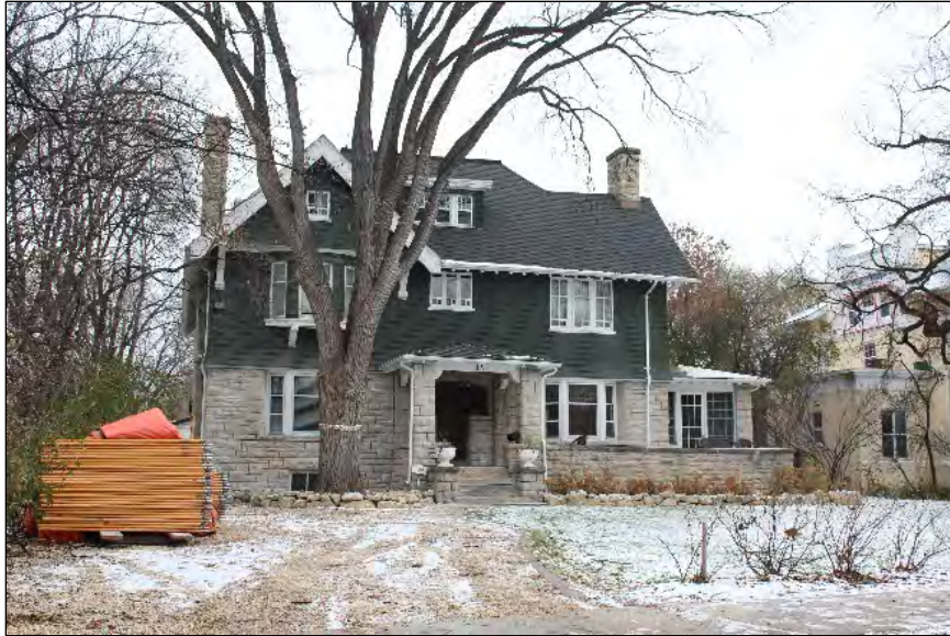
Heritage Building, Principal 14 Ruskin Row Built: 1909 Designer: J.D. Atchison Contractor: J.C. Allardice Style: Queen Anne Influences
