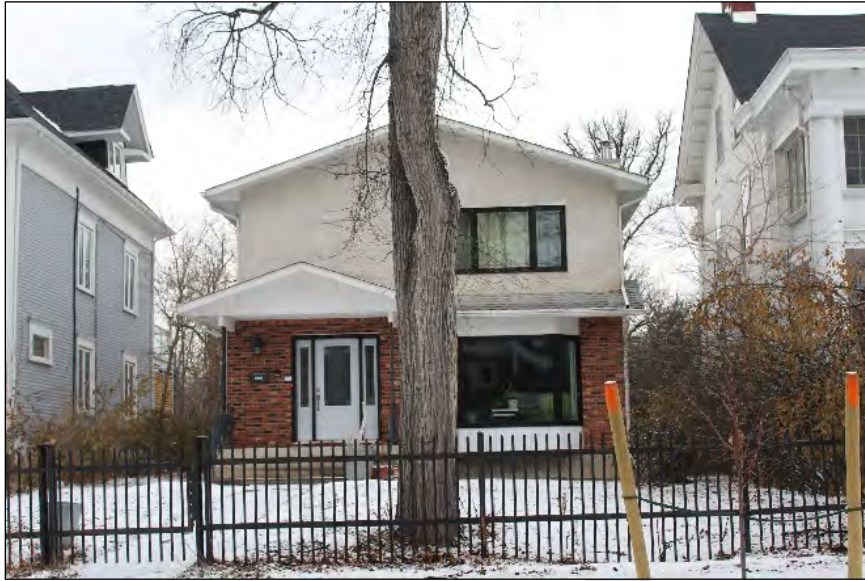
Non-Heritage Building 85 Kingsway Built: 1985 Designer: Unknown Contractor: Unknown
