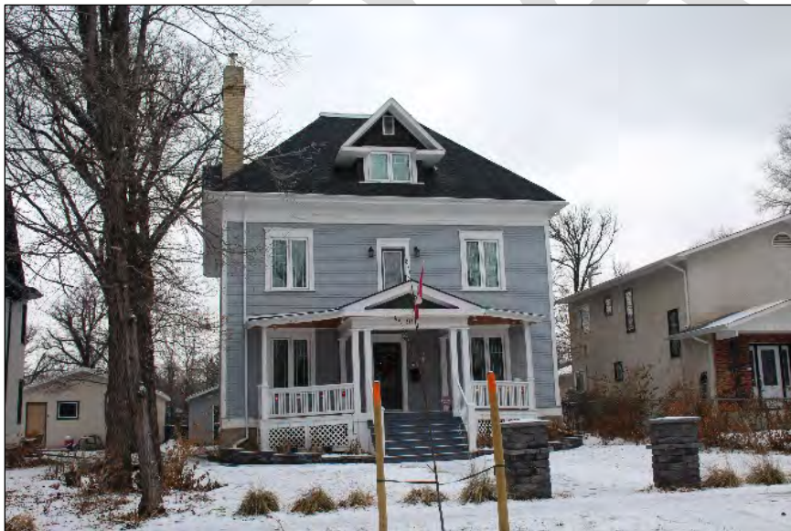
Heritage Building, Principal 91 Kingsway Built: 1905 Designer: J. Graham Contractor: J. Graham Style: Victorian Influences
