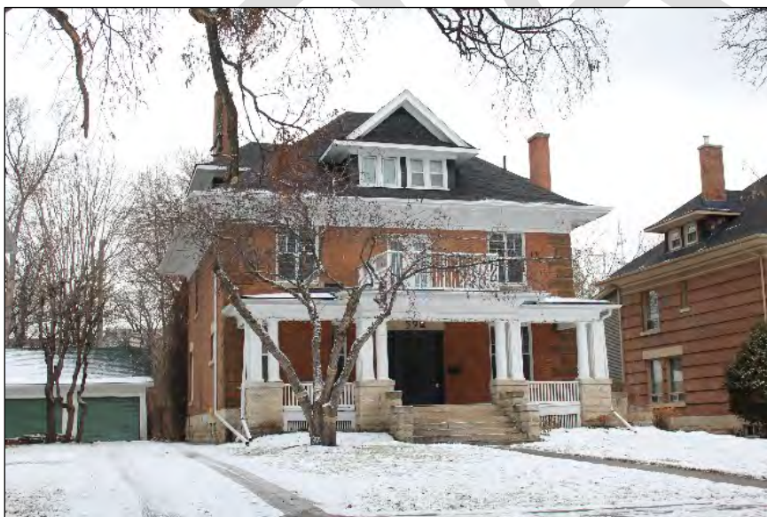
Heritage Building, Principal 59 Kingsway Built: 1908 Designer: R. Taylor (owner) Contractor: R. Taylor (owner) Style: Georgian Revival
