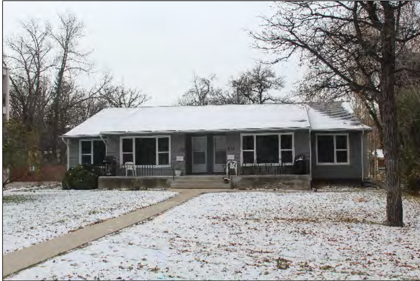
Non-Heritage Building 400 Wellington Crescent Built: 1953 Designer: Unnamed Contractor: Unnamed
