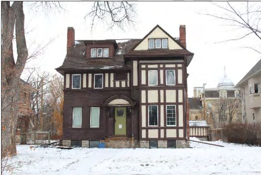
Heritage Building, Principal 47 Kingsway Built: 1906 Designer: Darling & Pearson Contractor: Davidson & Henderson Style: Tudor Revival
