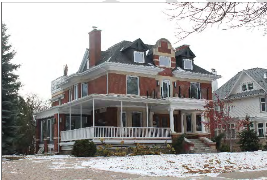
Heritage Building, Principal 54 Yale Avenue Built: 1908 Designer: W.W. Cross (owner) Contractor: W.W. Cross (owner) Style: Queen Anne
