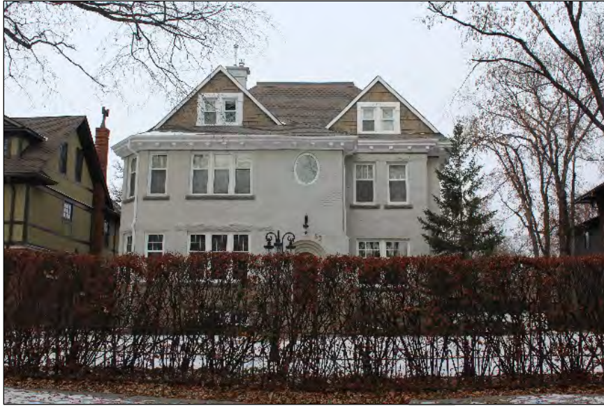
Heritage Building, Principal 53 Harvard Avenue Built: 1907 Designer: J.H.G. Russell Contractor: George Bray Style: Queen Anne Revival Influences
