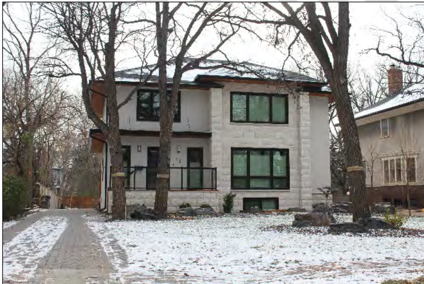
Non-Heritage Building 62 Harvard Avenue Built: 1929 (exterior alterations 2016) Designer: J.H. Saul (owner) Contractor: J.H. Saul (owner)
