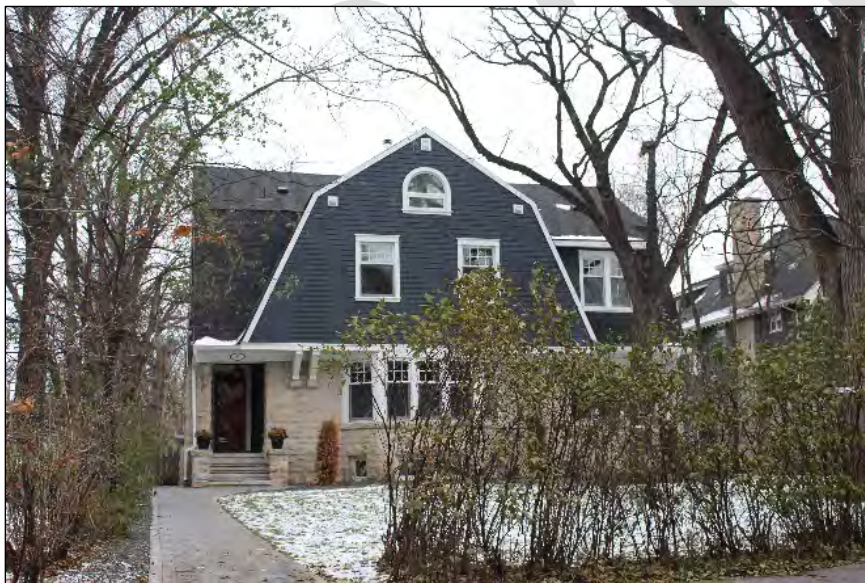
Heritage Building, Principal 16 Ruskin Row Built: 1908 Designer: J.D. Atchison Contractor: Davidson Brothers Style: Dutch Colonial
