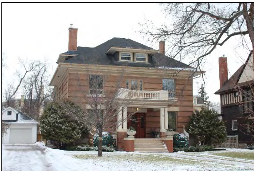
Heritage Building, Principal 53 Kingsway Built: 1908 Designer: R. Taylor (owner) Contractor: R. Taylor (owner) Style: Georgian Revival
