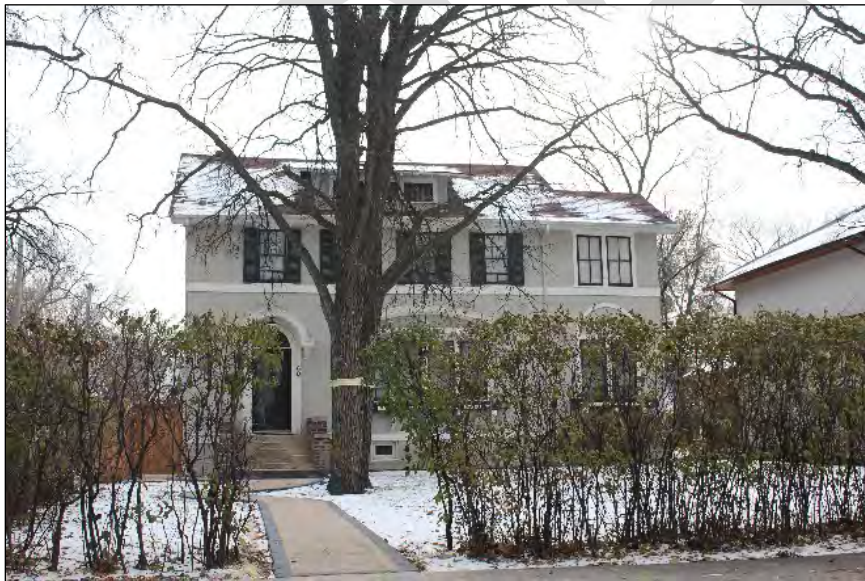
Heritage Building, Principal 60 Harvard Avenue Built: 1924 Designer: J.A. Fraser (owner) Contractor: J.A. Fraser (owner) Style: Georgian Revival Influences
