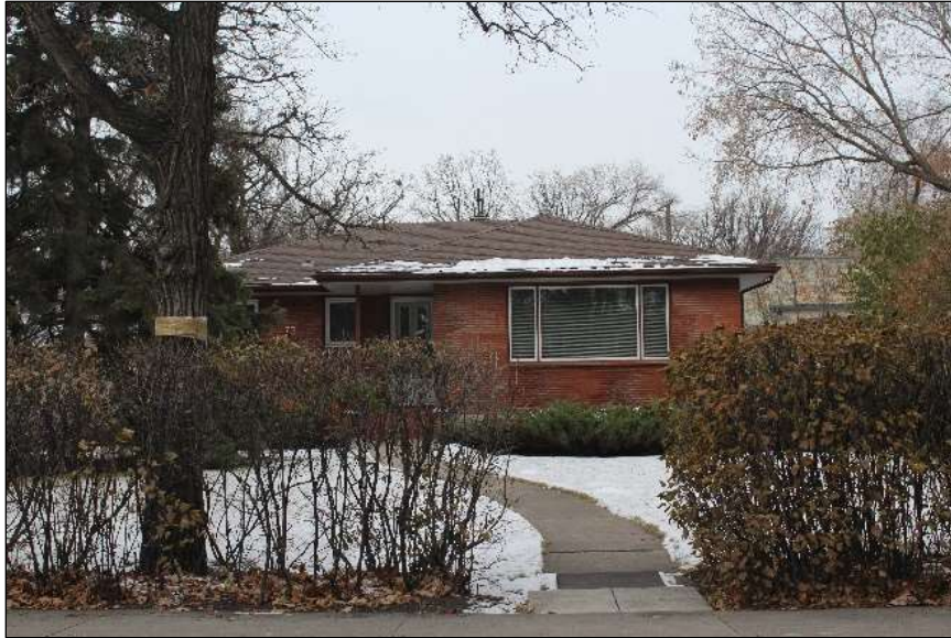
Non-Heritage Building 73 Harvard Avenue Built: 1953 Designer: Unknown Contractor: Parkin Brothers
