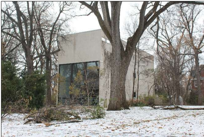
Principal Building, Heritage 2 Avonherst Street Built: 1974 Designer: Ron Keenberg/IKOY Contractor: Unknown Style: Late Modern/International Style Influences
