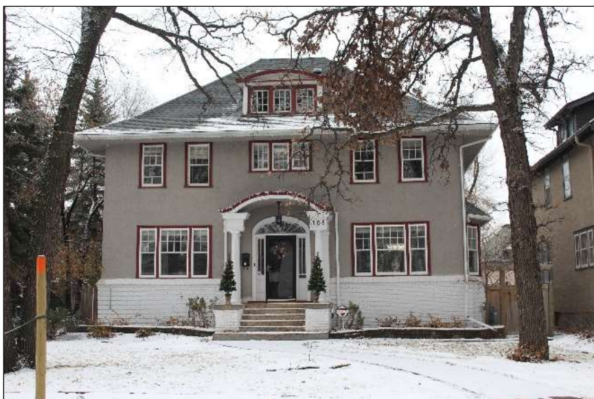
Heritage Building, Principal 108 Kingsway Built: 1926 Designer: W.P. Wallace (owner) Contractor: W.P. Wallace (owner) Style: Neoclassical Influences
