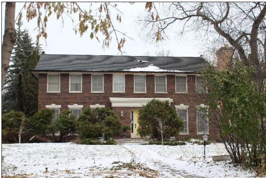
Non-Heritage Building 8 Ruskin Row Built: 1977 Designer: Unknown Contractor: Unknown
