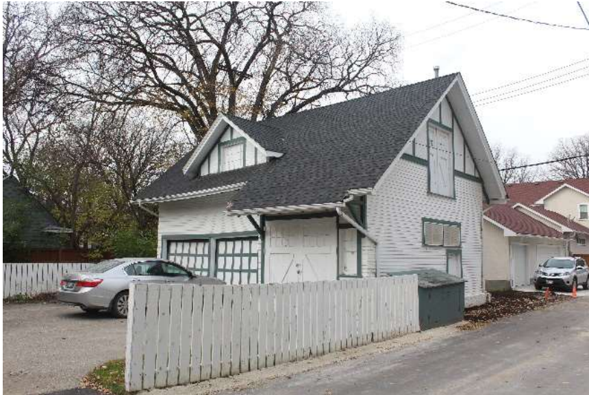
Heritage Building, Accessory 85 Yale Avenue
