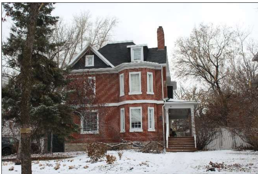
Heritage Building, Principal 73 Kingsway Built: 1906 Designer: J. Chisholm Contractor: Hinds & Mitchell Style: Queen Anne Revival
