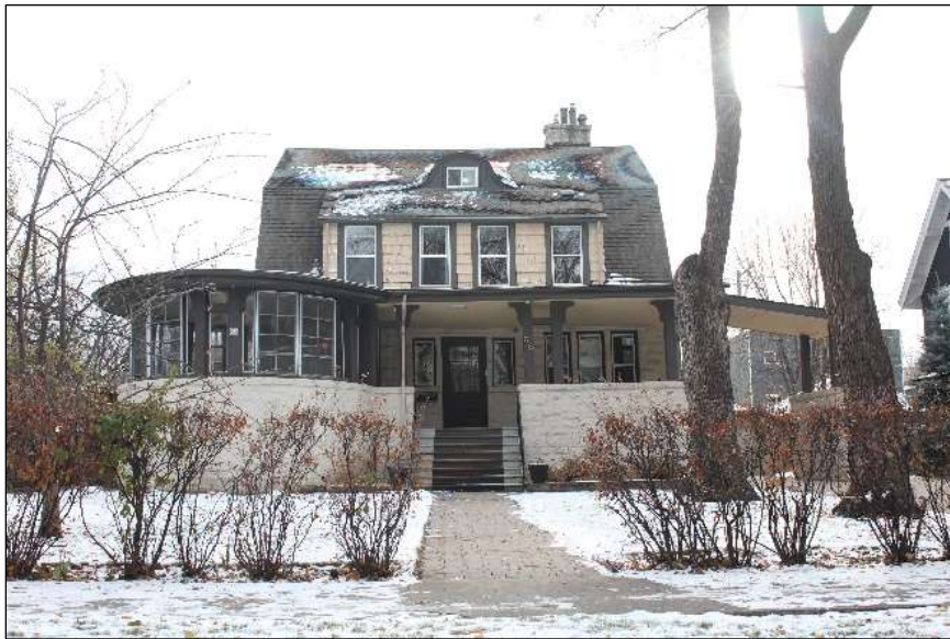
Heritage Building, Principal 68 Yale Avenue Built: 1906 Designer: H.B. Rugh Contractor: Gillis Fraser & McDonald Style: Dutch Colonial
