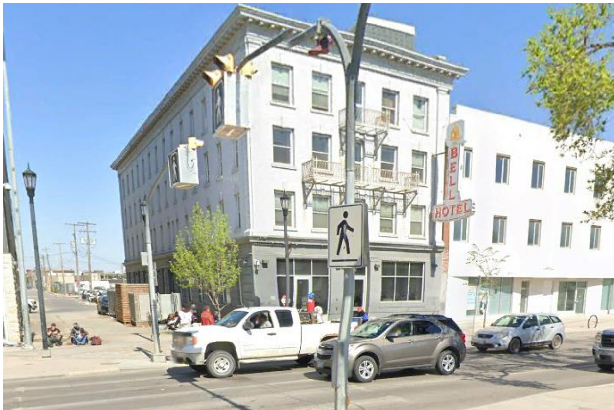
Figure 1: Google Street View image looking west towards Henry Avenue. Hope Alley is the open area between the two buildings.
