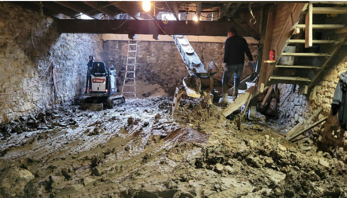
Excavating and stabilizing the basement (before)
