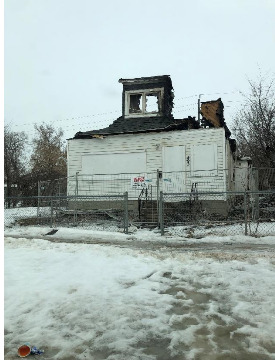
Located on Aberdeen Avenue. Spring 2025.
