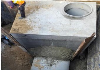
Land Drainage System - Pipe Installation
