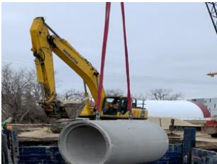
Land Drainage System - Piping
