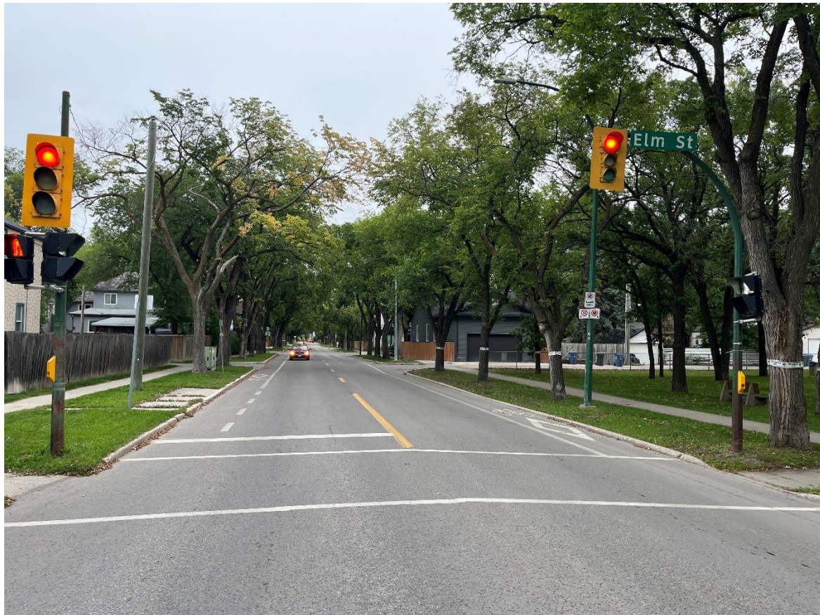
Figure 1 - Elm St and Grosvenor Ave Traffic Signal Aging Infrastructure
